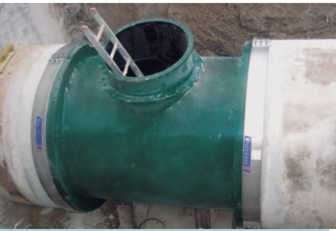
Fig. 5 / Installation of an inspection point in a large diameter pipe.
