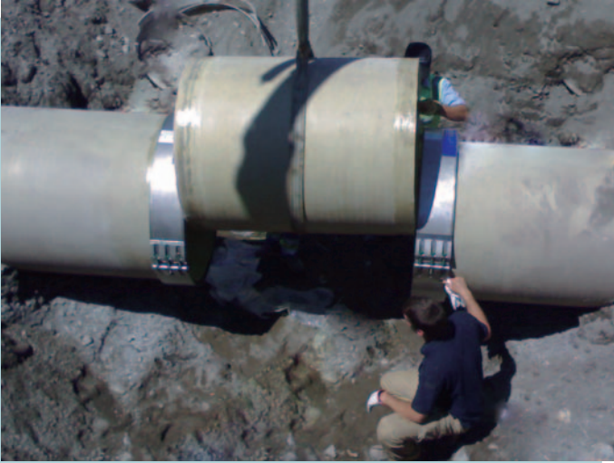
Fig. 1 / Fitting of an intermediate piece in a large diameter GRP pipe.
