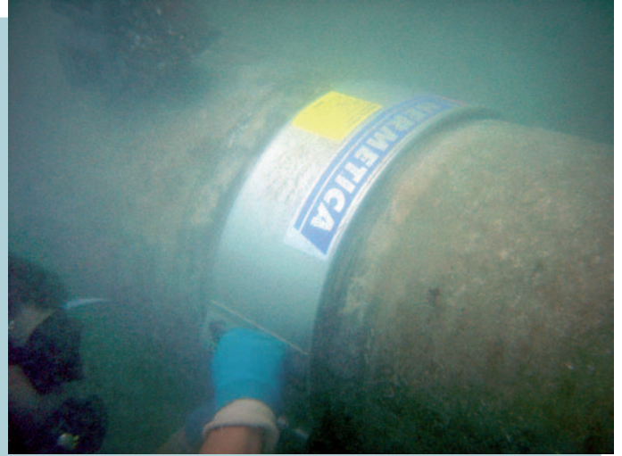
Fig. 2 / Underwater fitting. HERMETICA SF clamp made of Duplex stainless steel.
