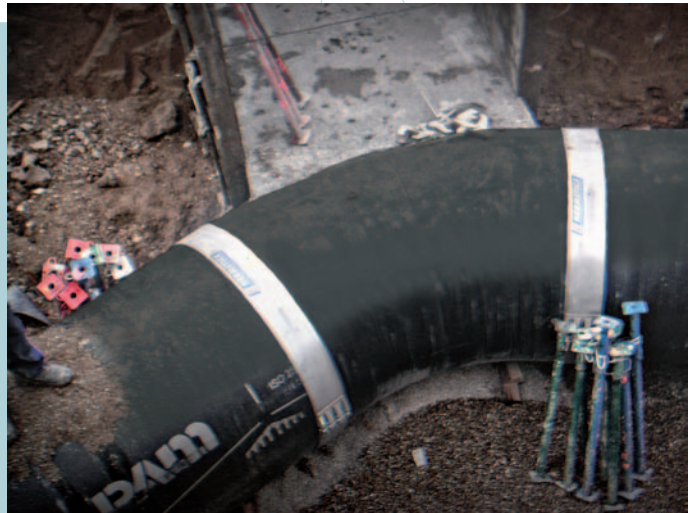
Fig. 4 / Assembly of cast iron pipes and accessories.
