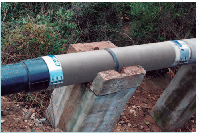
Fig. 6 / Repair of a pipe above ground, with different pipe material and diameters.
